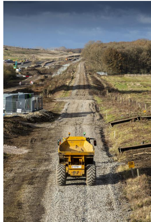
Plant operating on site in Finmere, December 2021.
