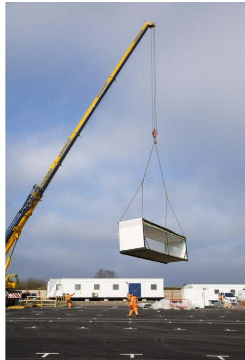
Temporary cabins being installed at one of our compounds, 2021.
